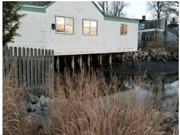
The stone rip-rap bulkheads shown in these photos are character-defining for the Wickford waterfront. Stone edges such as this should be retained whenever possible.
