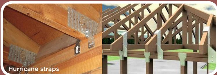
Code-plus techniques help fortify housing in areas prone to natural disasters such as hurricanes, floods, and wind- and snow-storms. Some examples include wind-and fire-resistant roofing, hurricane straps, impact and pressure resistant doors and windows, secure foundation, landscaping to reduce flood vulnerability.
