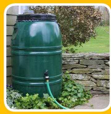
Rainwater harvesting using a rain barrel
